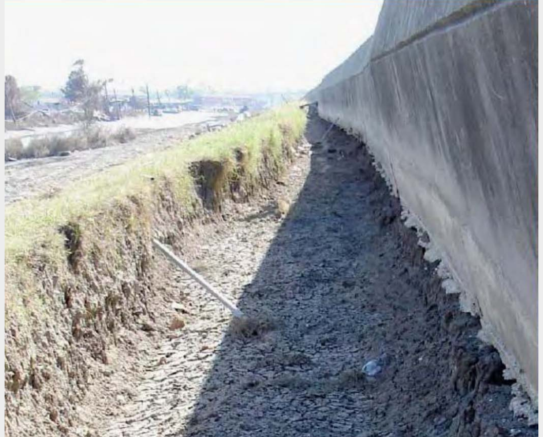
Scour and Erosion on the Protected Side of the IHNC Adjacent to the 9th Ward in the Vicinity of the South Breach
